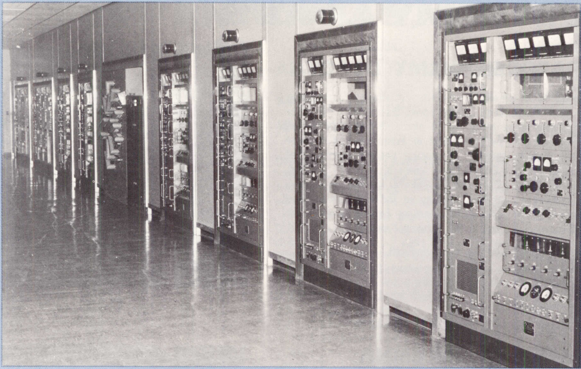
Interior view of a radio transmitter station installation using TMC 10 KW Synthesized transmitters.
