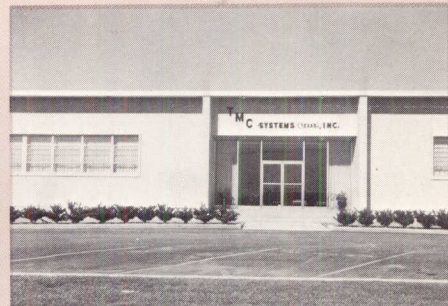
Office and Plant of TMC Systems (Texas) Inc., at Garland, Texas.
