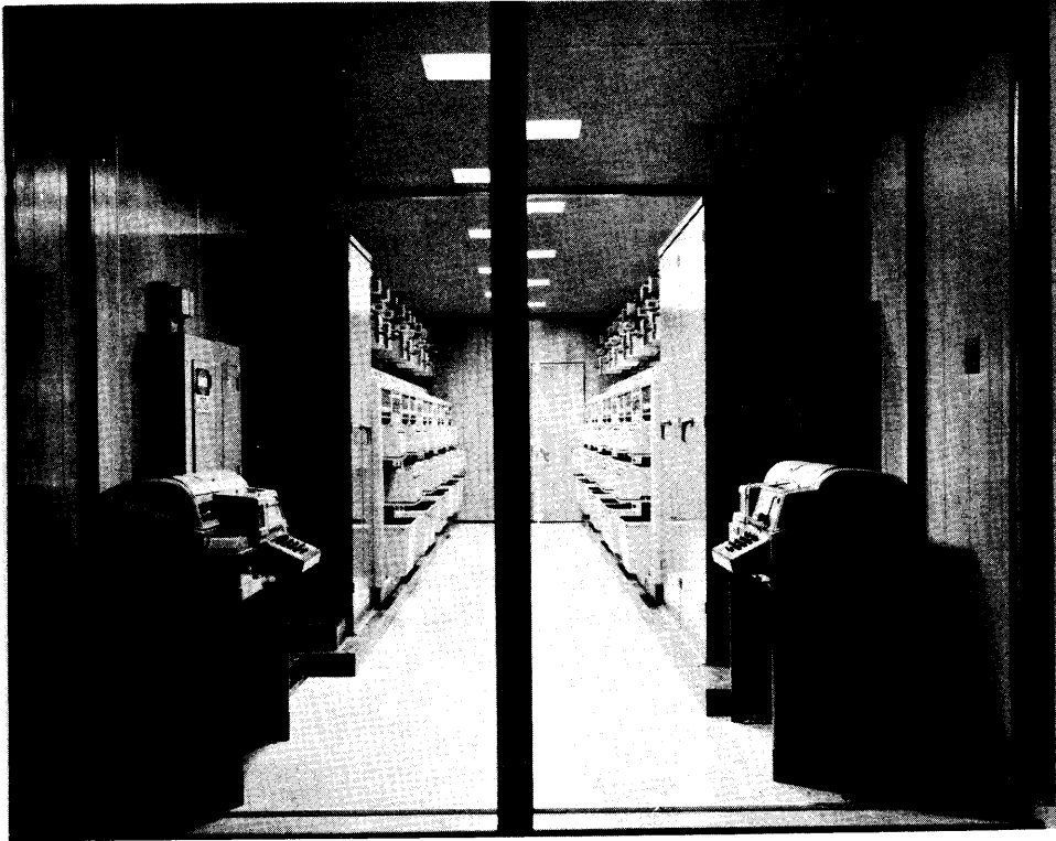
Figure 1-36. Teletype Central AN/TGC-19 (RJ2, Equipment Installation)
