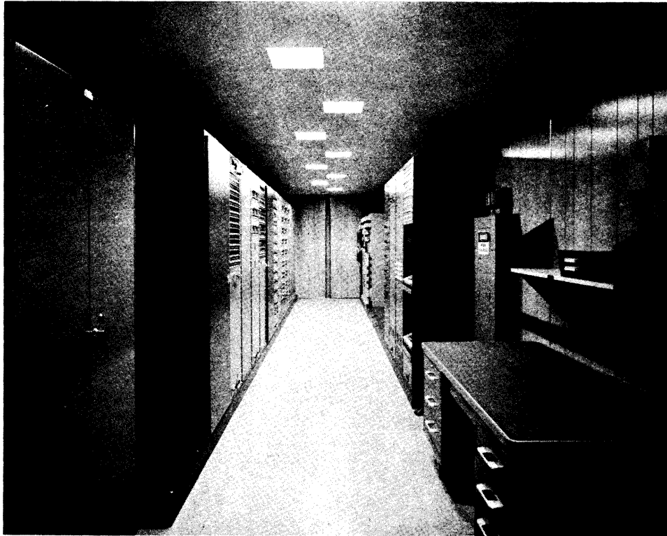
Figure 1-43. Control Monitor Group OA-4915/TST-2 (TC1, Equipment Installation)
