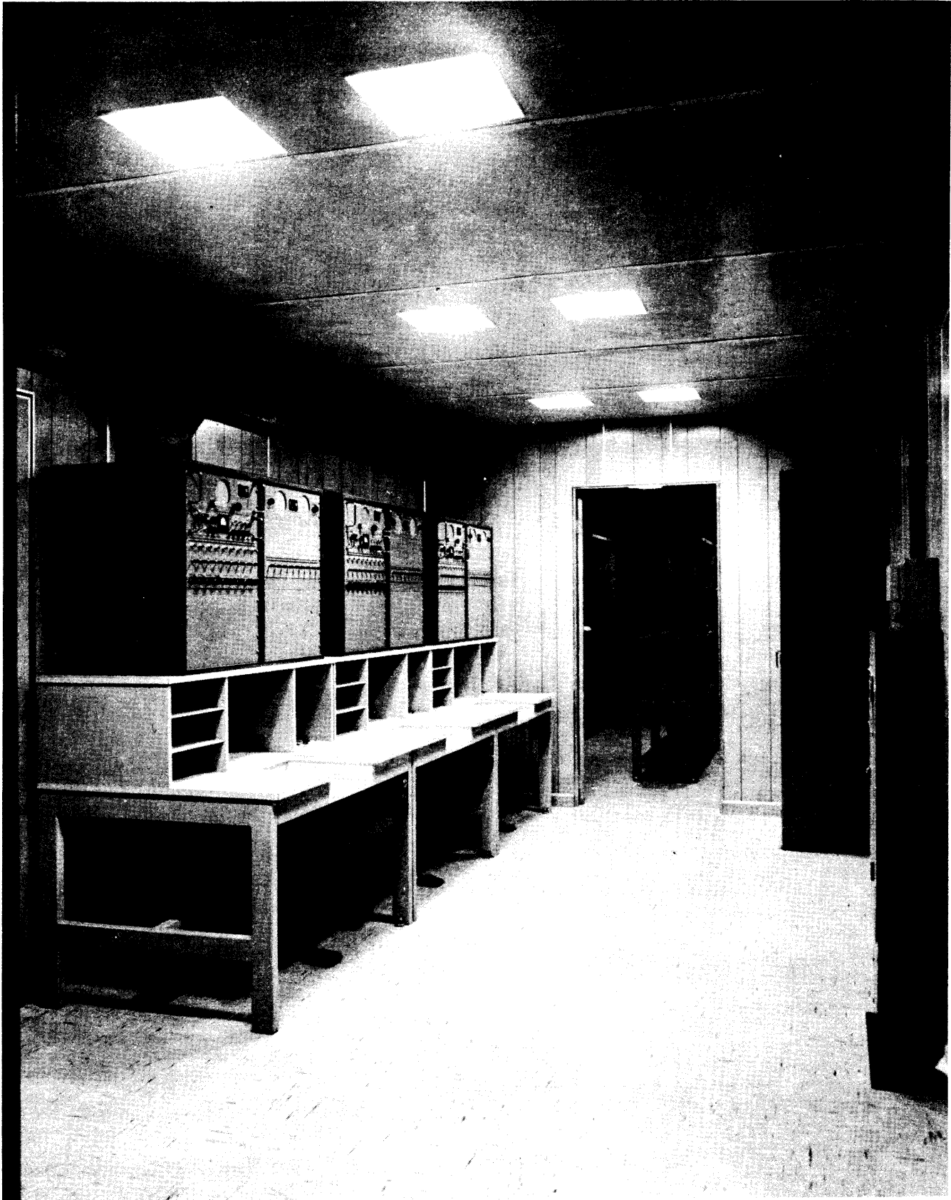
Figure 1-30. Control Monitor Group OA-4951/TSR-1 (RF3, Operations Area)
