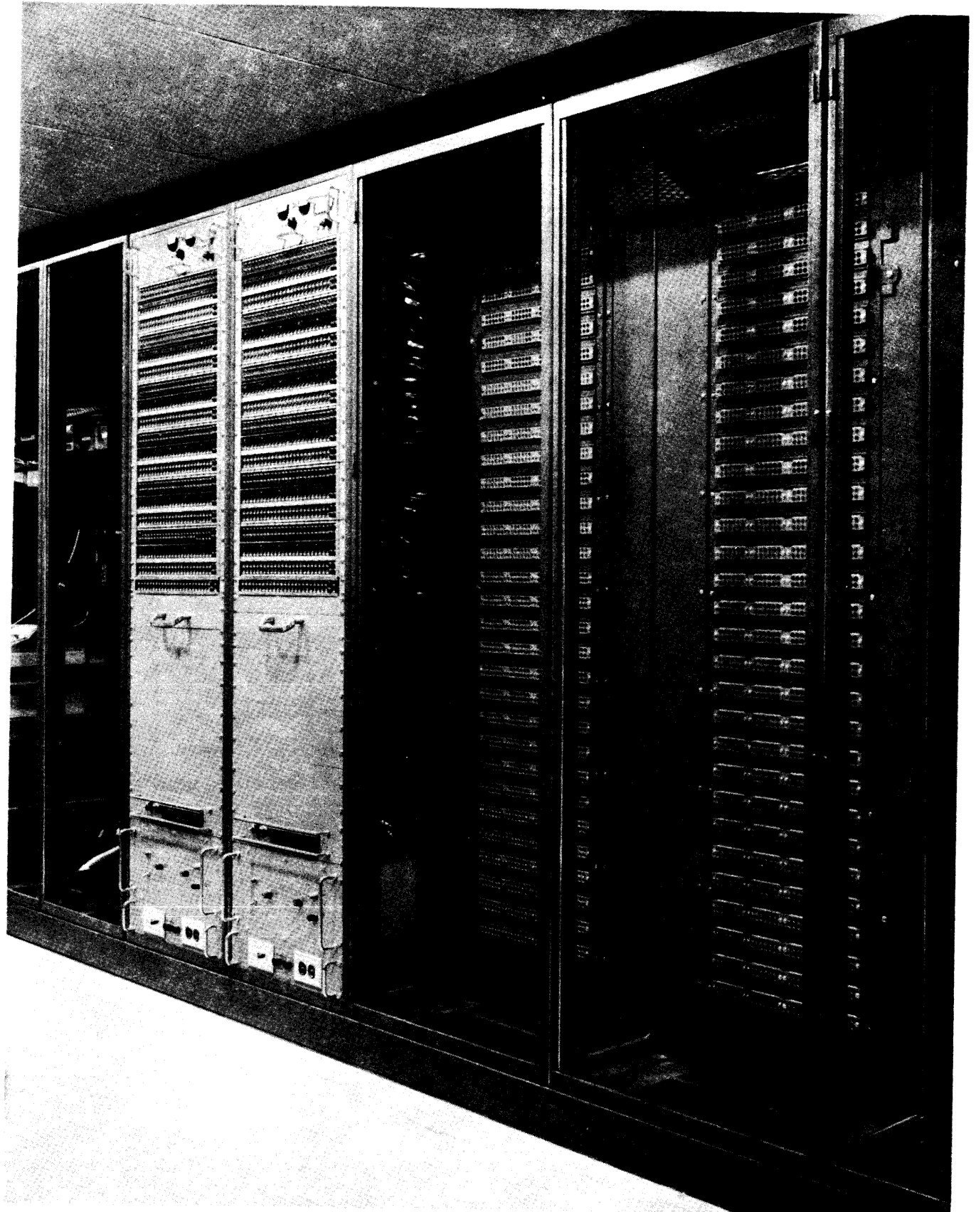
Figure 2-4. RED MDF Installation, Container RB1
