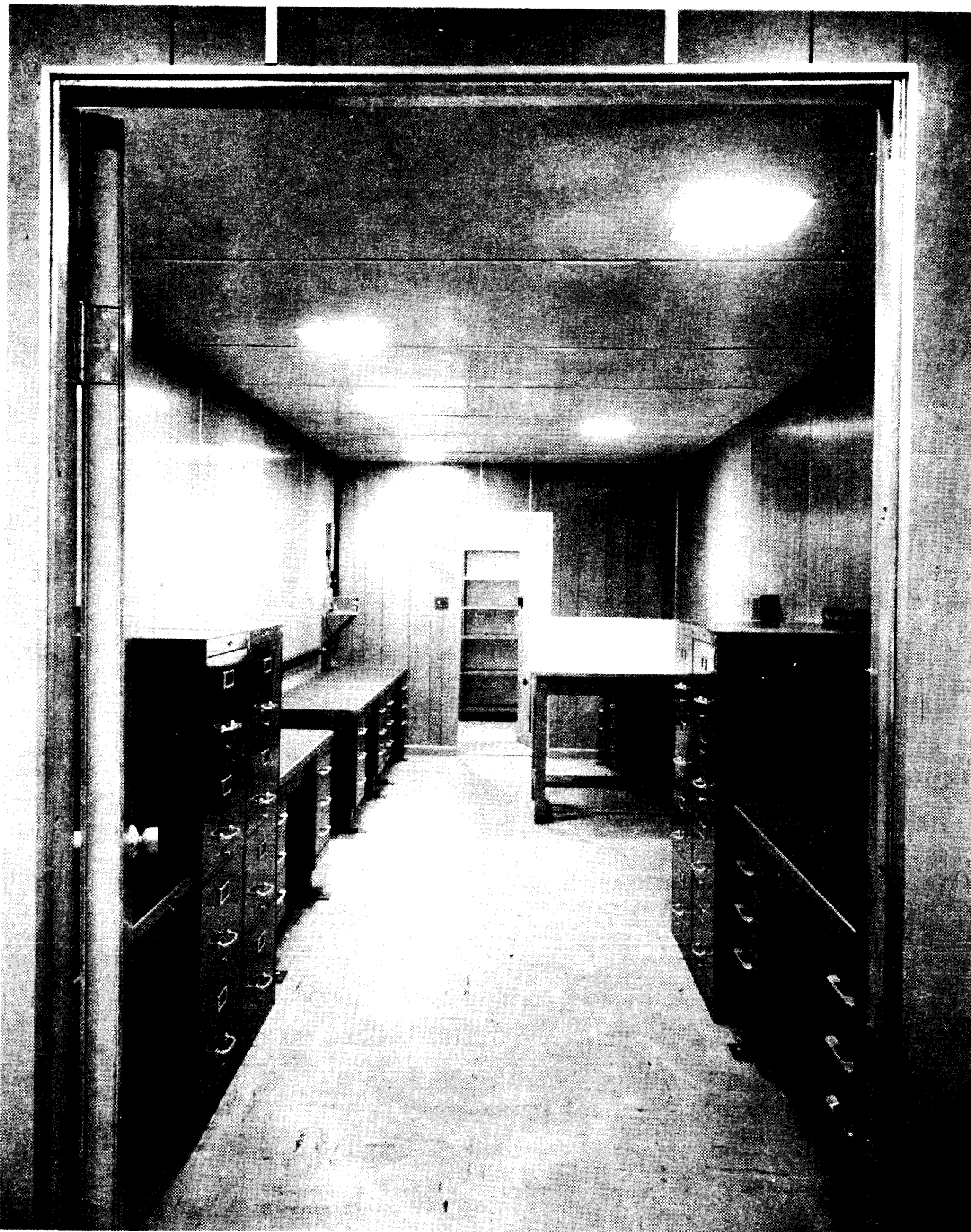
Figure 1-31. Receiving Central Group OA-4966/TSR-1 (RG1, Equipment Installation)
