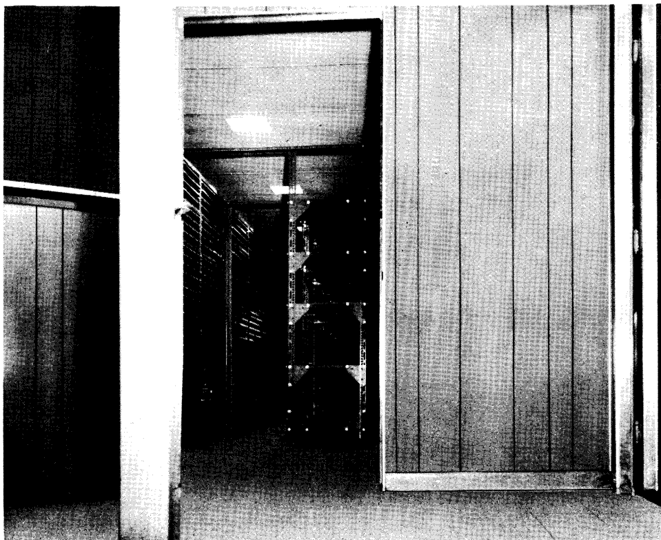
Figure 1-18. Supply Center OA-4942/TSR-1 (RD2, Rear Area)
