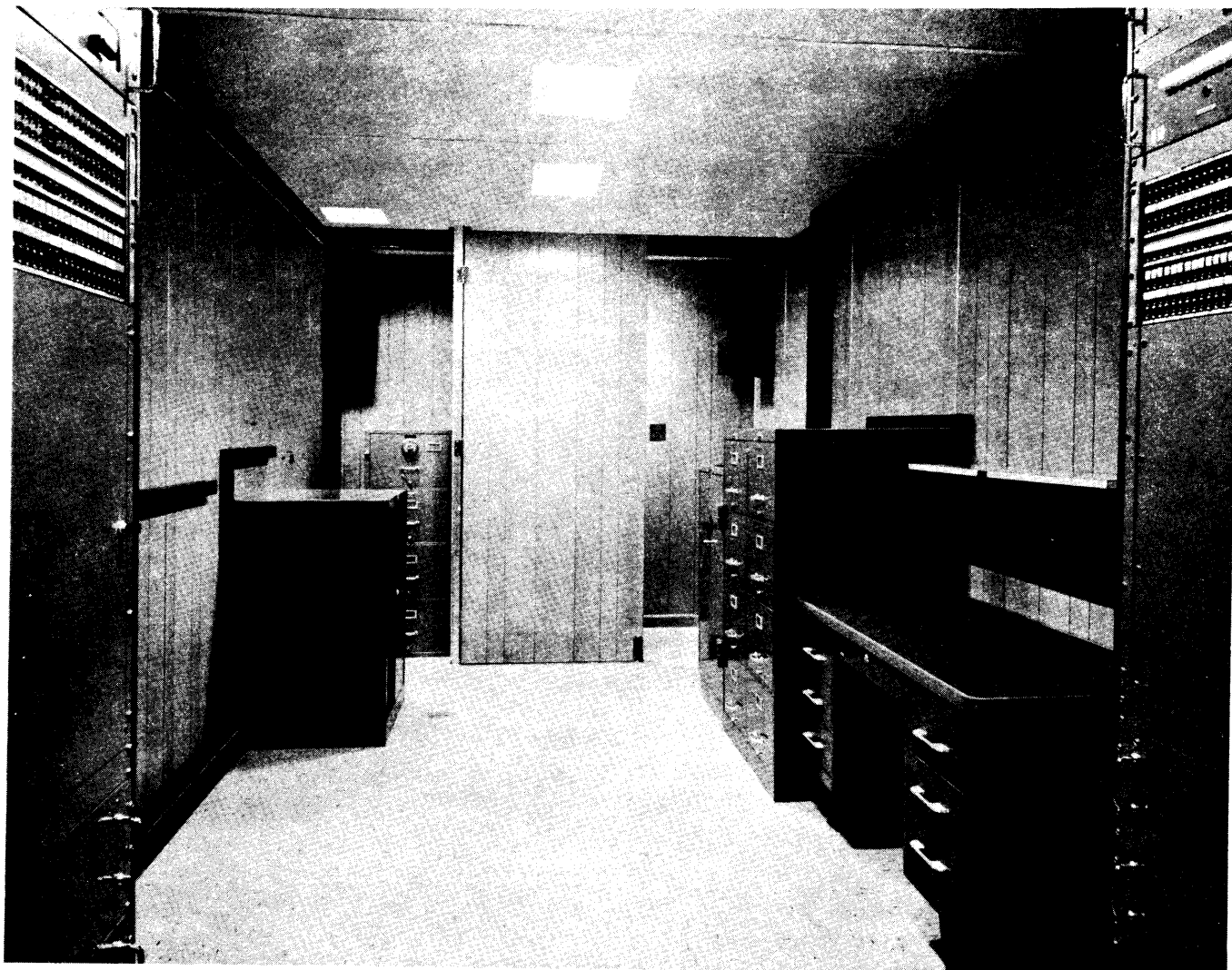
Figure 1-9. Receiving Central Group OA-7041/TSR-1 (RA3, Rear Area)
