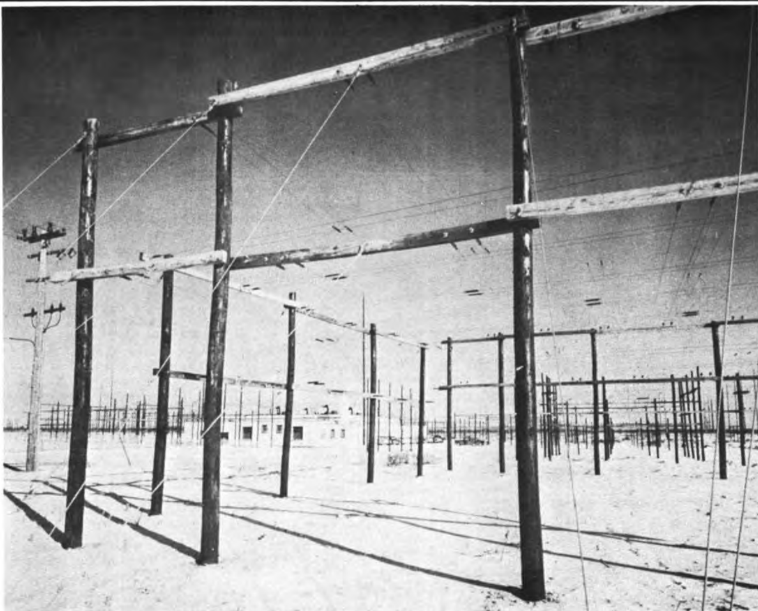
PART OF CENTEREACH DISTRIBUTION SYSTEM SUPPLYING MORE THAN 70 SEPARATE ANTENNAE.
